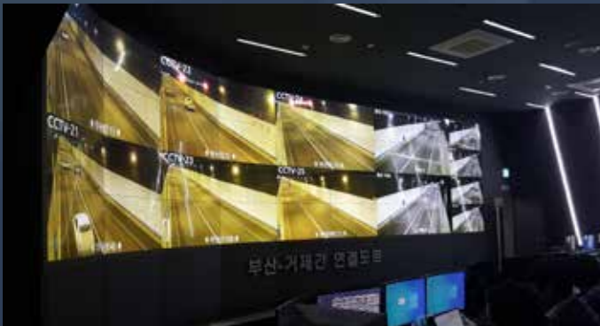
Hall-Integrated CCTV Monitoring Room, Geoje, Korea Application: security control and monitoring Configuration: 4x9 60" Visionpro® C series
