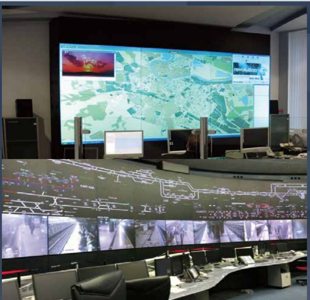
Hong Kong MTRC Super OCC : 3X33 80" DLP LED Cube with Digicom ARK Processors
