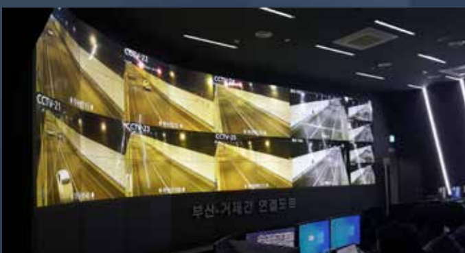
Hall-Integrated CCTV Monitoring Room, Geoje, Korea Application: security control and monitoring Configuration: 4x9 60" Visionpro® E series
